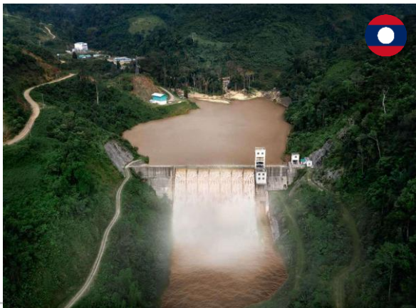
Hydro Power (2 Sites)
